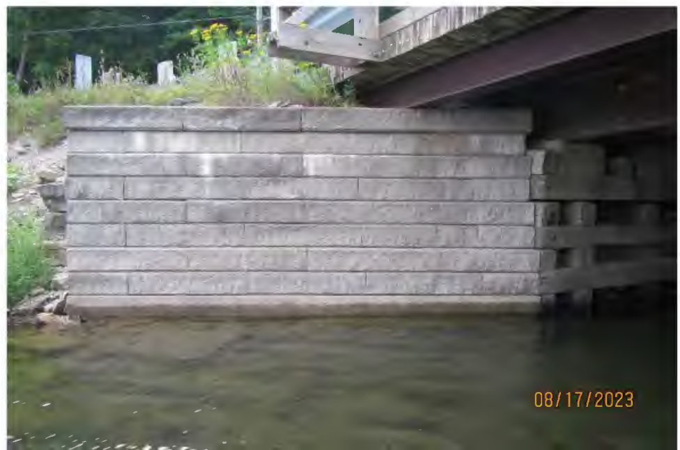
Photo 4 – Northeast wingwall (Typical)
