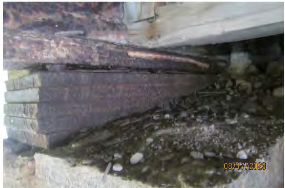
Photo 5 – West abutment shim plates at south bearing
