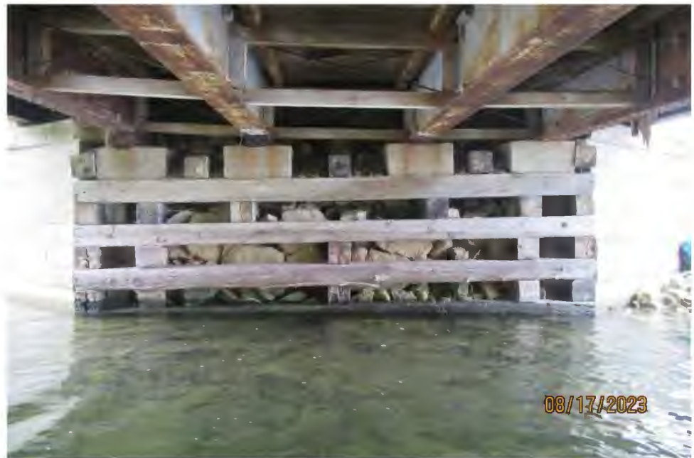
Photo 3 – West Abutment Elevation
