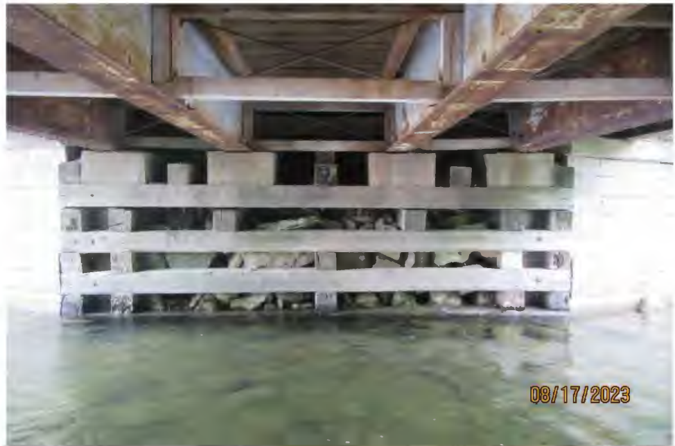
Photo 2 – East Abutment Elevation
