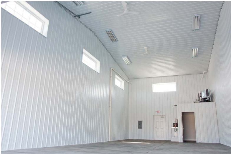
Figure 15 – Interior metal liner panel
