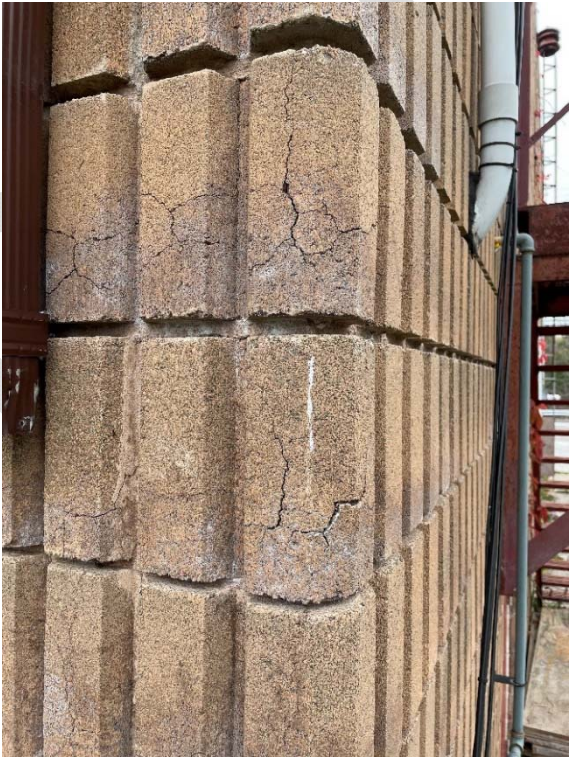
Figure 12 – Typical Exterior Masonry Condition
