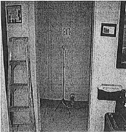
Photograph 1 Assessment sample BTWN-001-23-10-18 collected in the east portion of the office.
